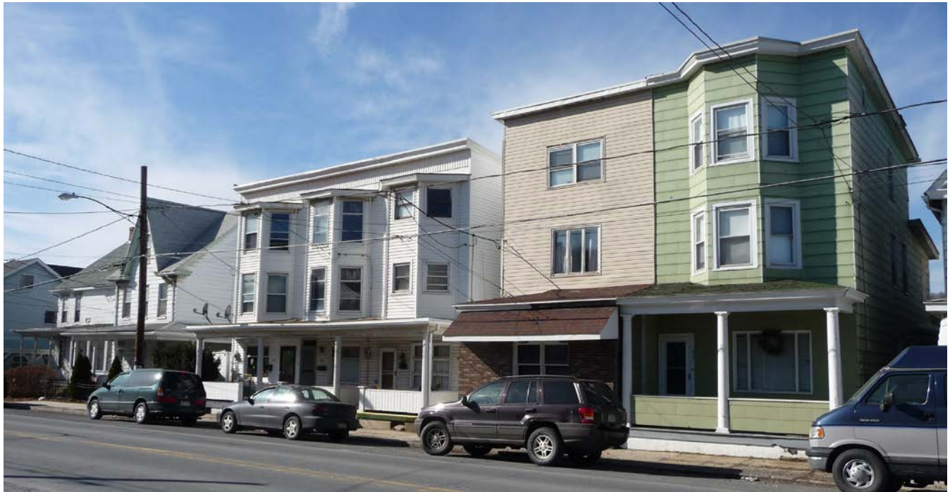
Figure #2: Representative example of vernacular duplex and row houses, East Bertsch Street facing northwest.
